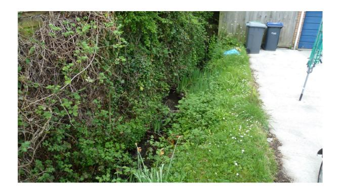
My calculations indicate that the open watercourse has a capacity of 2.3 cubic metres per second (2,300 litres per second). I measured a fall of 3.5% by placing my iPhone on the kerb line because the watercourse slope is similar to the road slope but physically measured the other dimensions.
